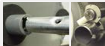
INSERT TUBES & TURN TOWARD AIRFLOW
